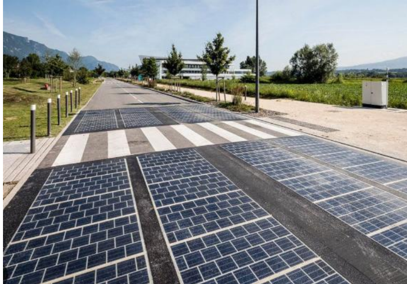
Figure 2.0: Solar Powered Roads
